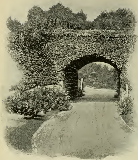
Bridge in Delaware Park.
